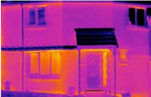
Figure 11a: Thermographic image of the front of the Masonry House.
