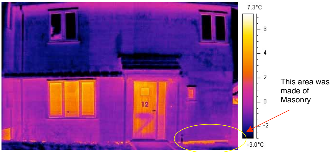
Figure 6: Thermographic image which represents the front elevation of the Hemp House as shown in Figure 5: Colour graduation represents temperature scale of -3°C to 7.3°C.
