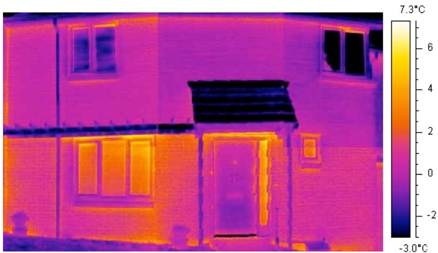
Figure 2: Thermographic image which represents the front elevation of the Masonry House as shown in Figure 1: Colour graduation represents temperature scale of -3^{\circ}\text{C} to 7.3^{\circ}\text{C} .
