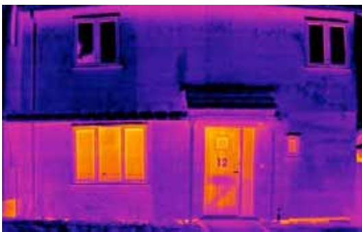
Figure 11c: Thermographic image of the front of Hemp House.
