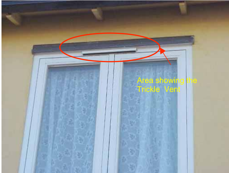
Figure 9: This photo showed the area where there was heat loss from the trickle ventilation (at the back window of the Hemp House).
