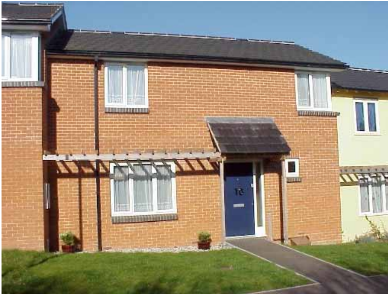
Figure 1: Front elevation of the Masonry House at No.10 Teasel Close, Haverhill, Suffolk.
