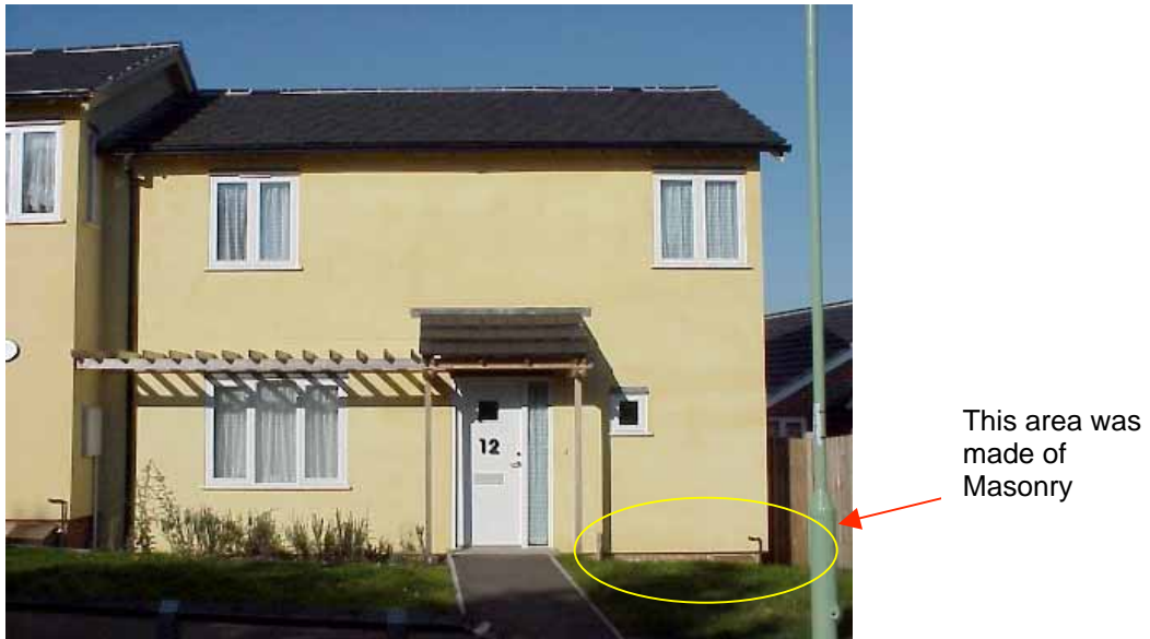
Figure 5: Front elevation of the Hemp House at No.12 Teasel Close, Haverhill, Suffolk.
