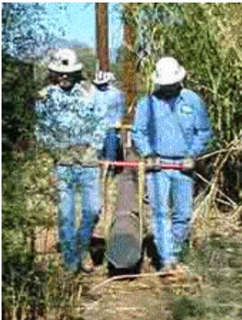
**Remote installation of a composite pole (Powertrusion)**
