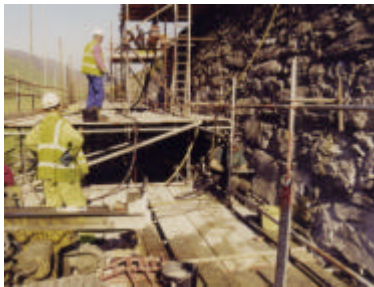
Wall stabilisation with soil nails
