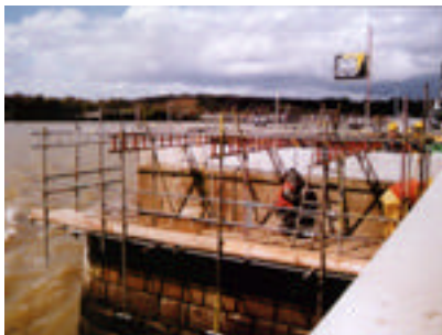
Reinforcement of dock wall
