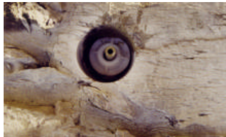
Wall stabilisation with soil nails
