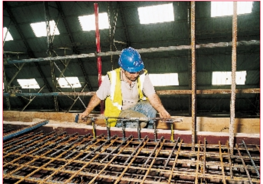
Figure 1: Fixing prefabricated shear reinforcement at Cardington
