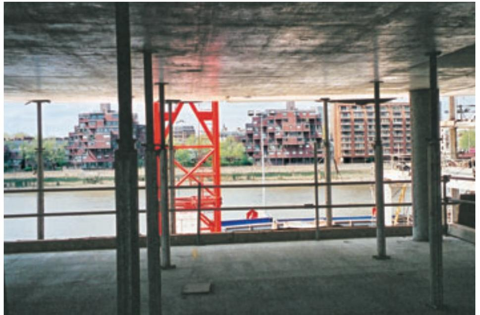
Figure 1: Backpropping installed at St George Wharf
