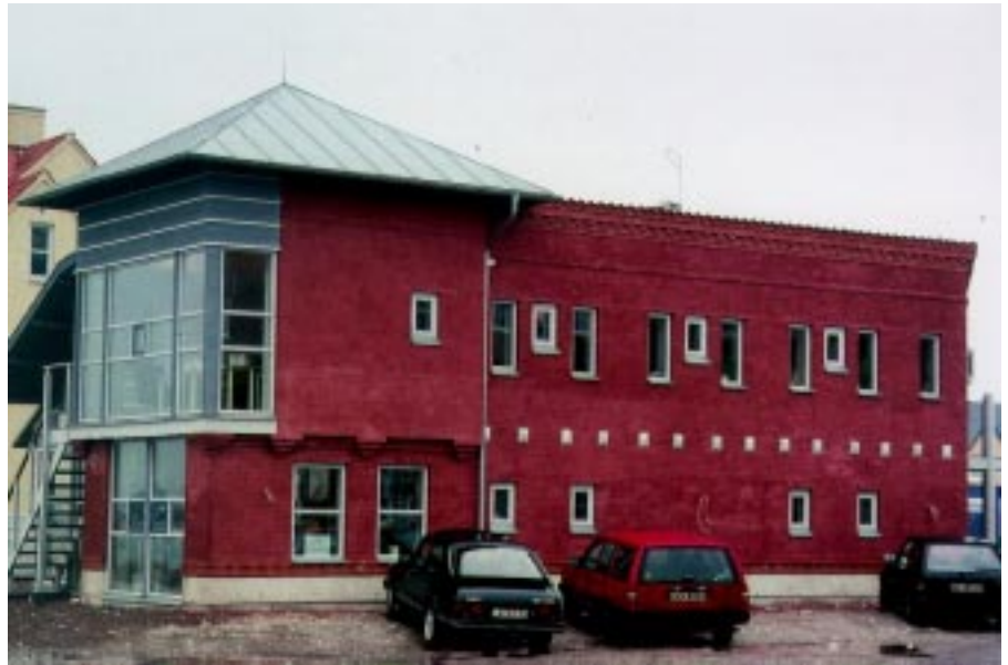
Figure 1: View of the Tage Moller Building, Malmo
