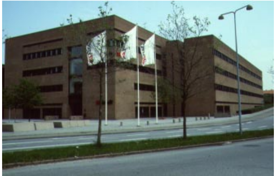
Figure 1: View Showing Main Building in Foreground and Office Block 2 on Right
