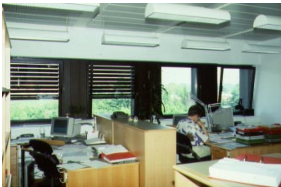
Figure 4: Interior of an Office Showing Exterior Blinds and Multi-Position Windows
