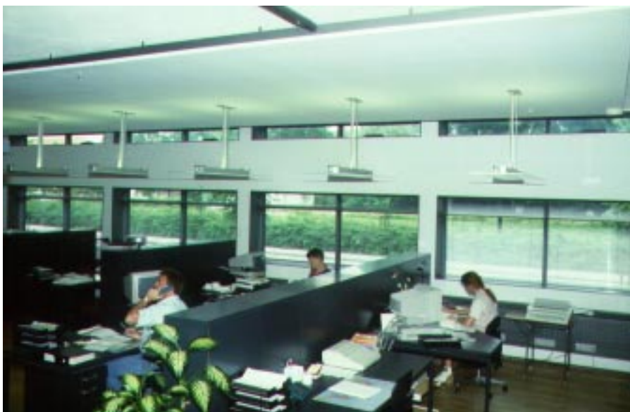
Figure 4: View From Inside an Office Illustrating Narrow Window Bands Above the Main Windows
