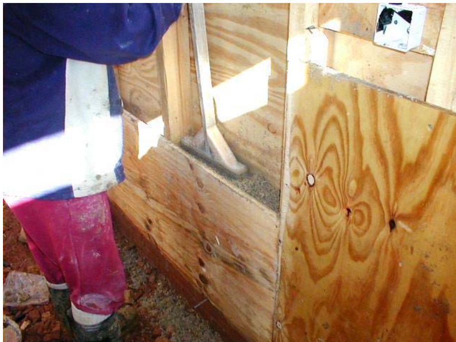
Figure 2 Tamping the hemp/lime into the shuttering
