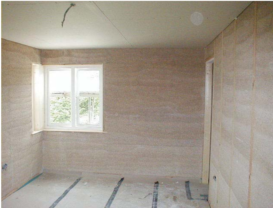
Figure 3 Ground floor interior near the completion of the 'shell'
