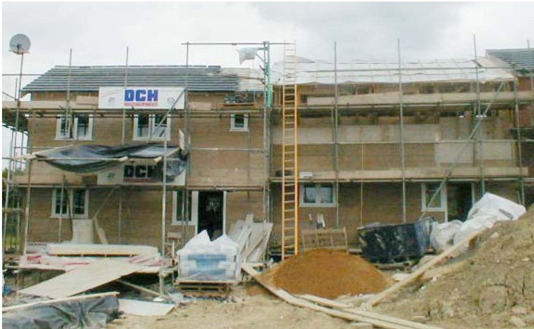
Figure 5. Hemp Homes on 12.06.01
