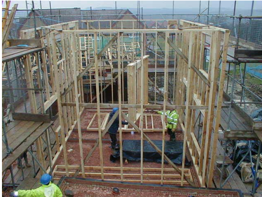
Figure 2 Tamping the hemp/lime into the shuttering
