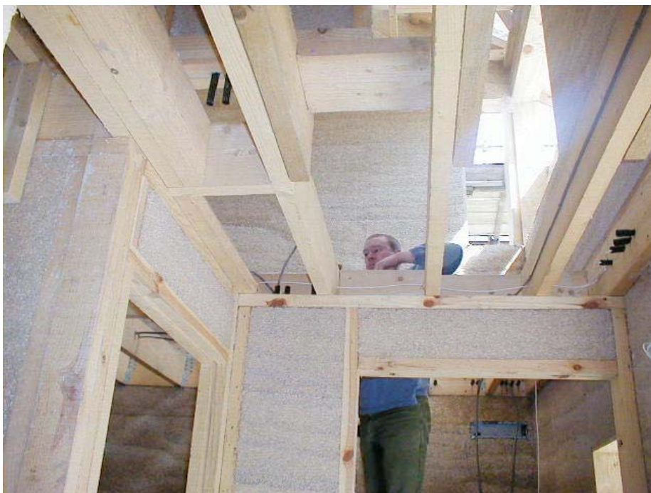
Figure 4 Wiring and construction of interior partitions
