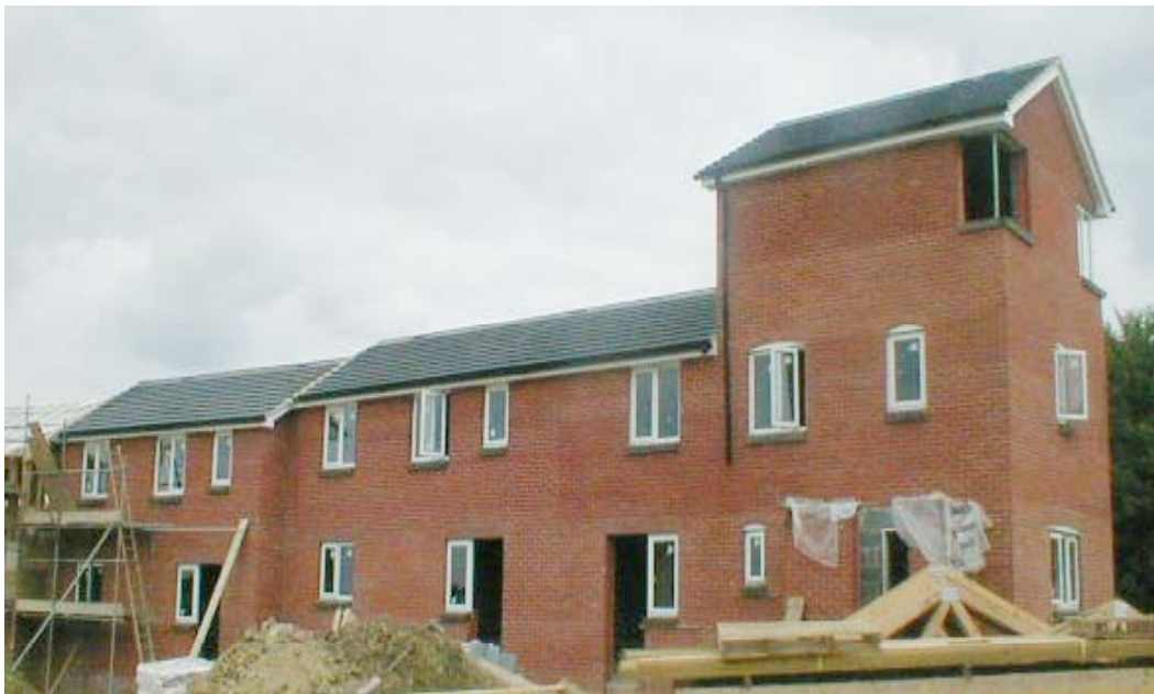
Figure 6. Traditional houses nearing completion
