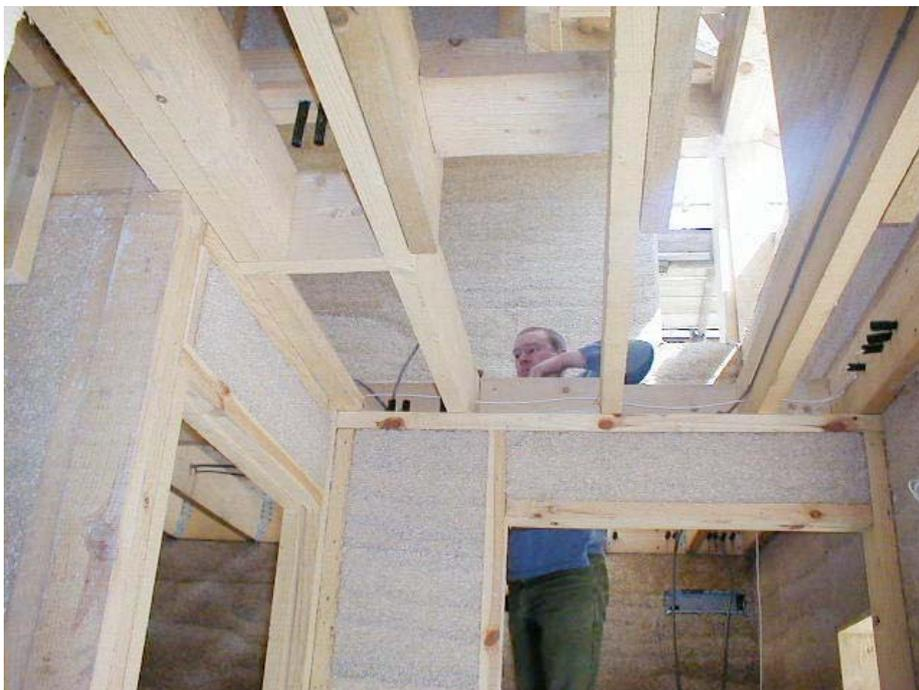
**Figure 4** Wiring and construction of interior partitions
