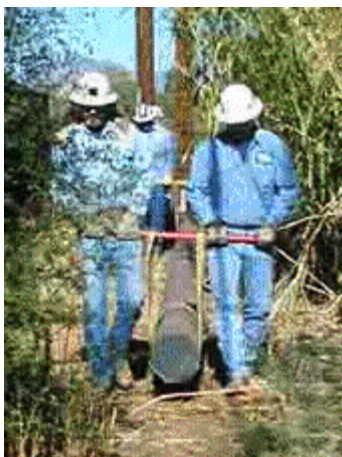
Remote installation of a composite pole (Powertrusion)
