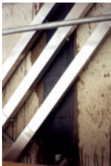
Strengthening of concrete walls at nuclear power station
