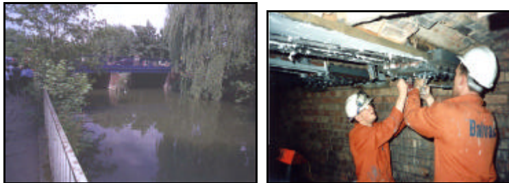
Strengthening of Hythe Bridge, Oxfordshire
