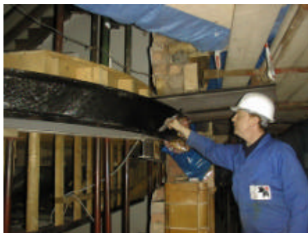
Laminating curved beam
