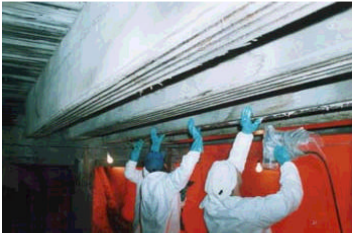
Installing glass epoxy rods in timber beams
