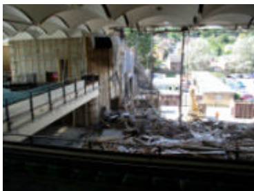
Demolition scrap– all GRP internal roofing went to landfill
