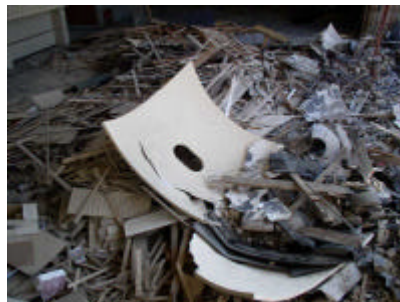
Demolition scrap– all GRP internal roofing went to landfill
