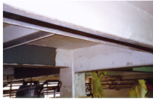
Strengthening of beams in a building
