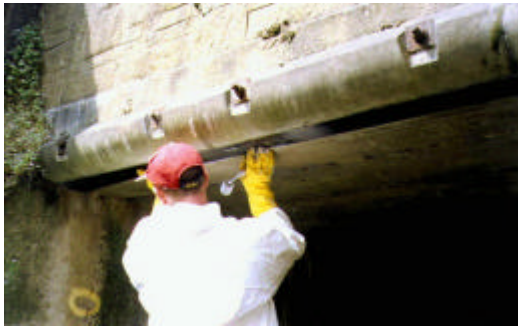
Strengthening of a bridge
