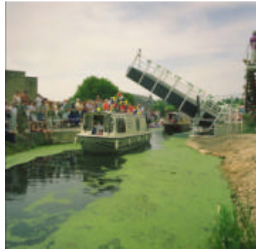
Bonds Mill Lift Bridge
