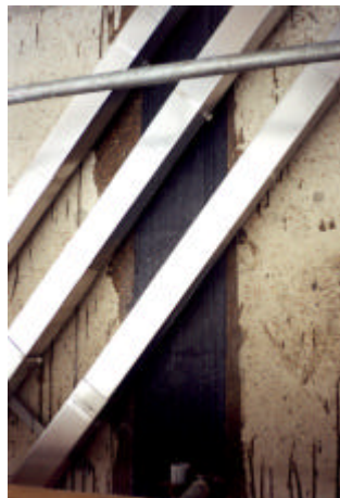
Strengthening of Tower at Nuclear Power Station
