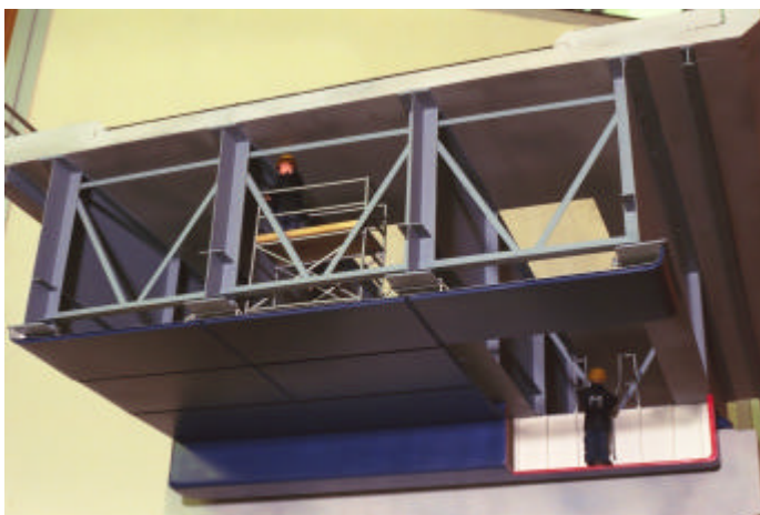
Figure 4 : Concept of Bridge Enclosure for access, via A19 Tees Viaduct, NE England
