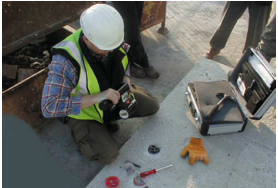
Figure 1: Lok test being carried out on a floor slab
