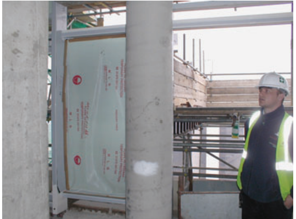
Figure 1: The improved finish from the use of self-compacting concrete for vertical elements
