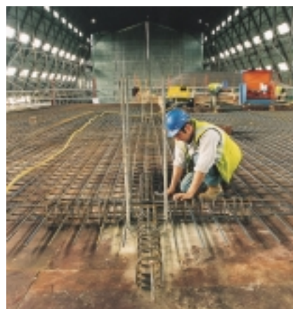
Figure 7: ACI shear stirrups were prefabricated at Cardington
