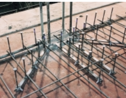
Figure 5: Stud rails at Cardington
